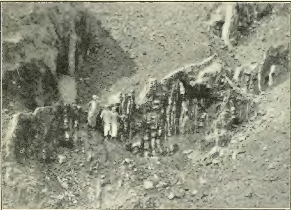
NATIVE OPEN-CUT WORKING ON WOLFRAMITE VEINS.
